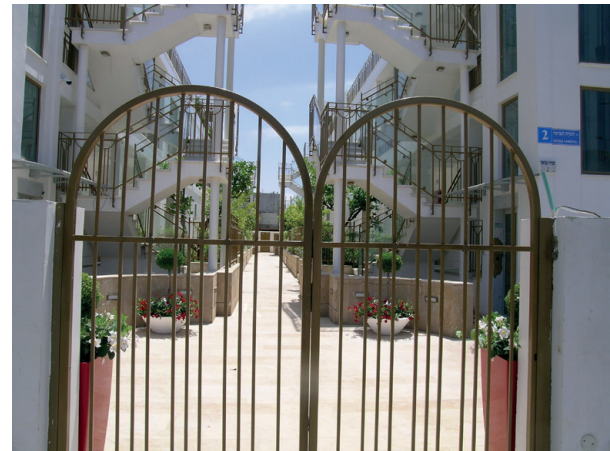
Figure 21. N. Portugali, Entrance Gate- the threshold connecting the site and the street.
