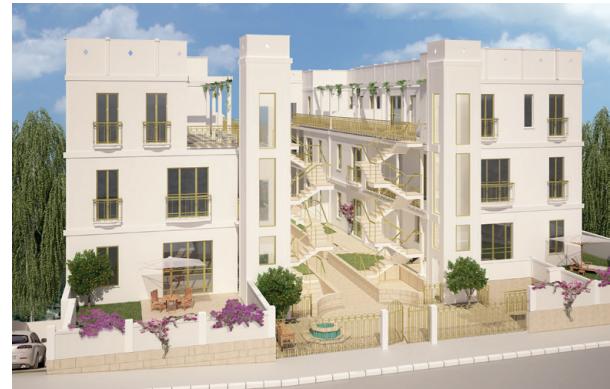
Figure 20. N. Portugali, Entrance Gate- the threshold connecting the site and the street.
